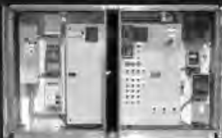
Pad Mounted Control Packages
