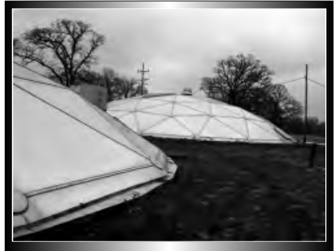
Aluminum Covered Trickling Filters
