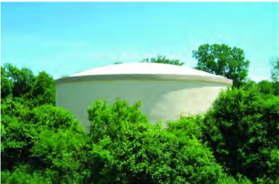
1.0 MG Natgun water tank for the Village of Rosin, IL. Engineering by Robinson Engineering, Ltd., South Holland, IL.
