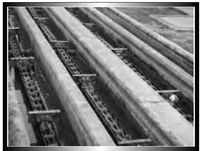
Three-channel grit removal
