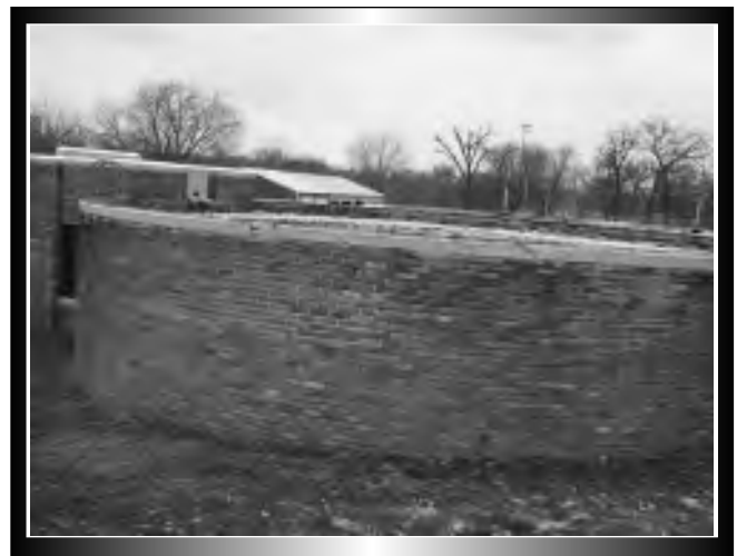
Old anaerobic digester with roof missing
